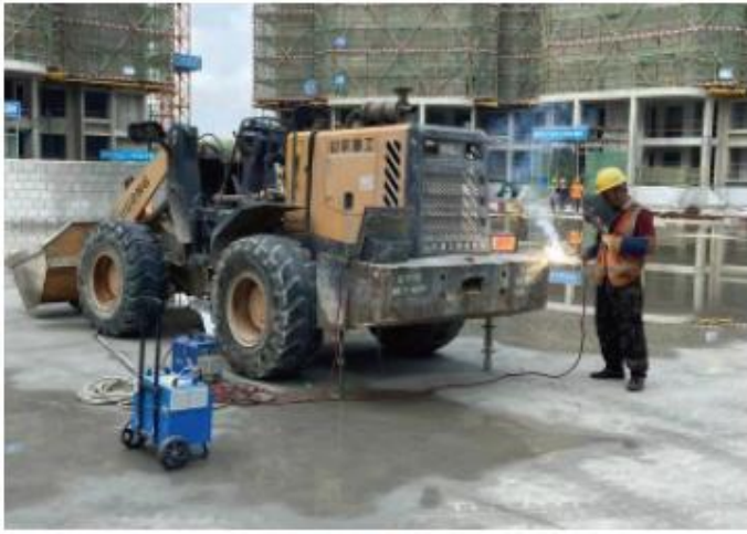
Power for construction works
