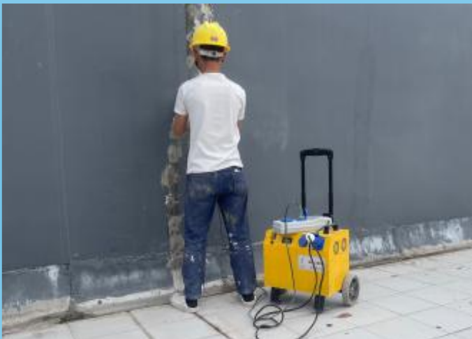
Power for tunnel engineering
